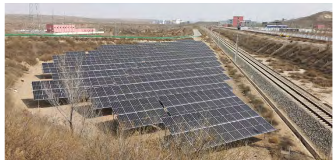
Fig.2 PV connected into traction power supply
